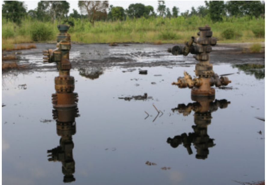
Creaking infrastructure in the Niger delta
